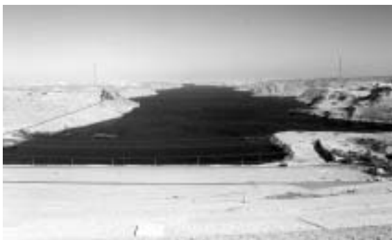
Aswan High Dam, Egypt
